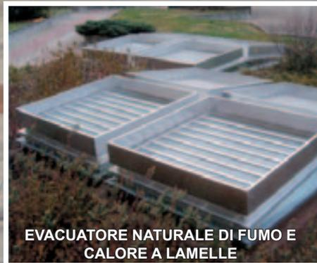
EVACUATORE NATURALE DI FUMO E CALORE A LAMELLE
